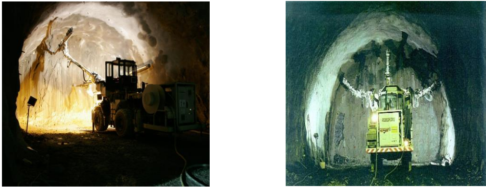
Figure II-1: perforation des trous
