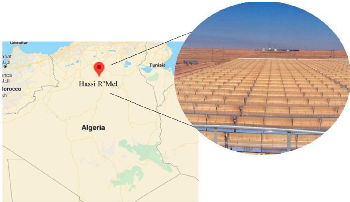
Figure I.15. Station CSP de Hassi R'mel.
